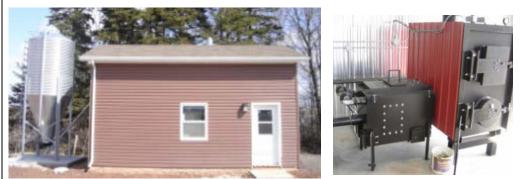
A small building (with outside fuel hopper) houses a 75 kW cereal grain combustion unit made by Grovewood Heat of Little York, PEI.
