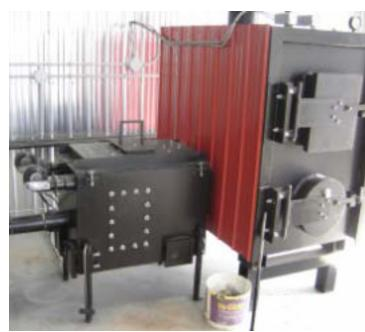
*A small building (with outside fuel hopper) houses a 75 kW cereal grain combustion unit made by Grovewood Heat of Little York, PEI.*
