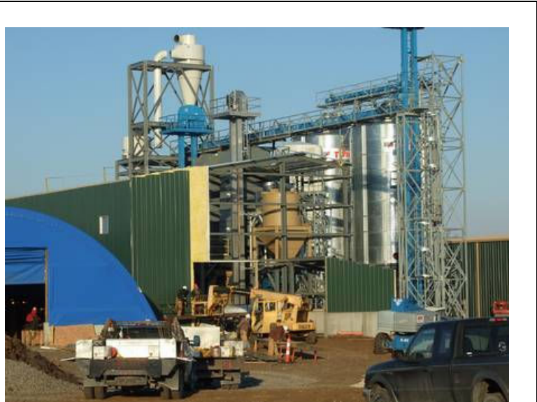
Show Me Energy Cooperative processing facility under construction ( www.goshowmeenenergy.com )
