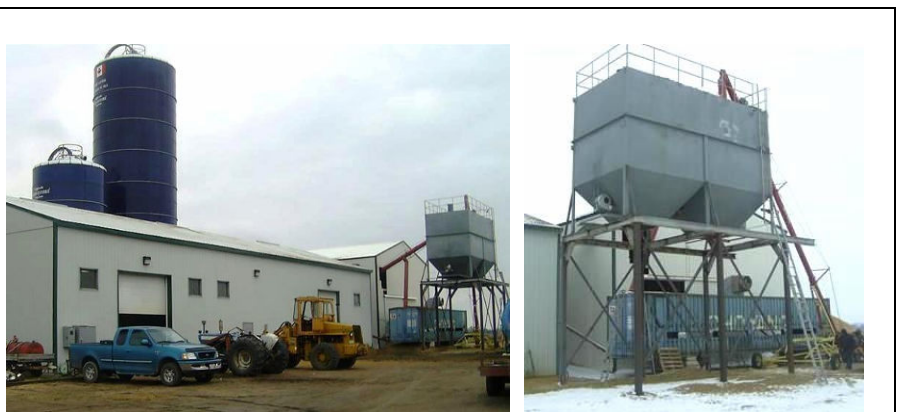
In 2005, Prairie Bioenergy became the first Canadian producer of densified crop residues for energy. Their biomass cubes are loaded into an overhead bin for bulk loading into trucks
