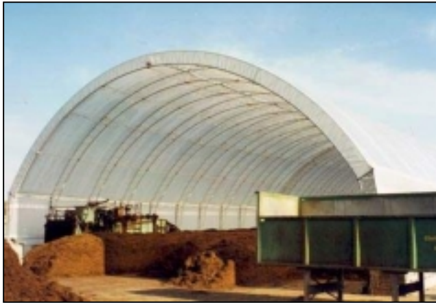
Photo 3.8 Single arch, woven fabric shelter can be used for bulk storage
