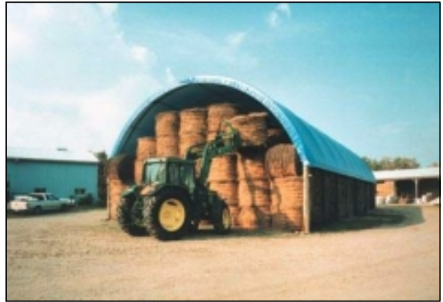
Photo 3.9. Single arch, woven fabric shelter for storing bales
