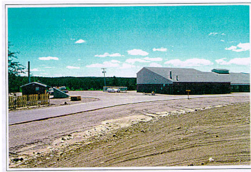
New school at Armstrong, Ontario, with chip-fired boilerhouse on the left.
